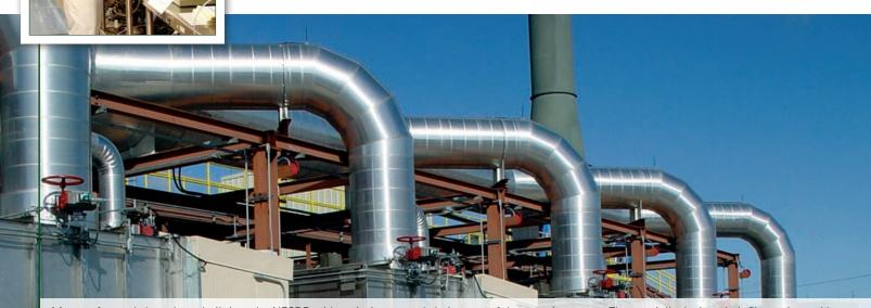
Many safeguards have been built into the NECDF, with emission controls being one of the most important. The specially designed air filters pictured here scrub the air to remove particulates and pollutants in order to meet state and federal clean air standards.
