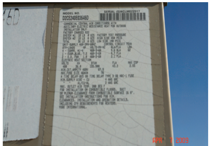
Name plate for warehouse HVAC unit
