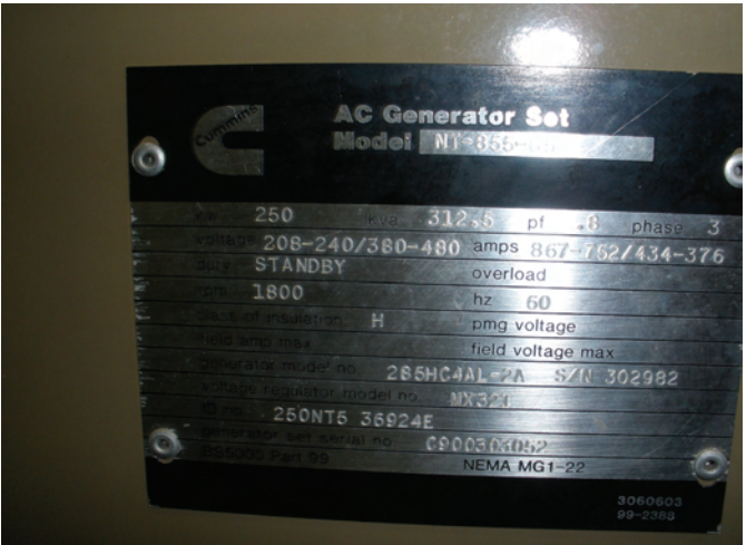
250KW Cummins Generator
