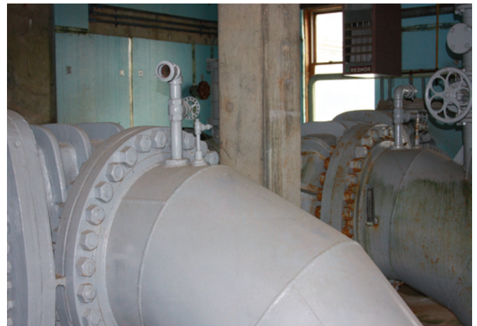
Inlet House: 2 each 36" inlet pipes
