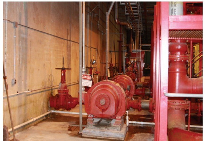
Fire suppression water supply pumps (3)
